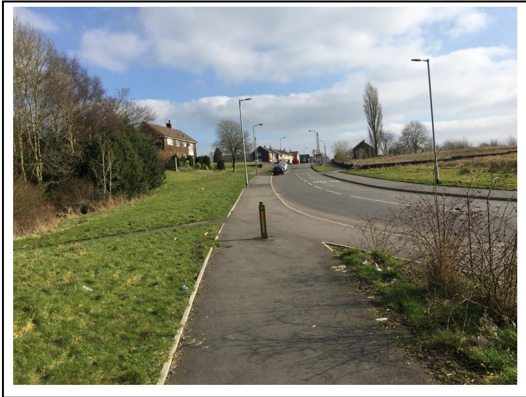
Photo 3 – view looking east along Hattersley Road West
