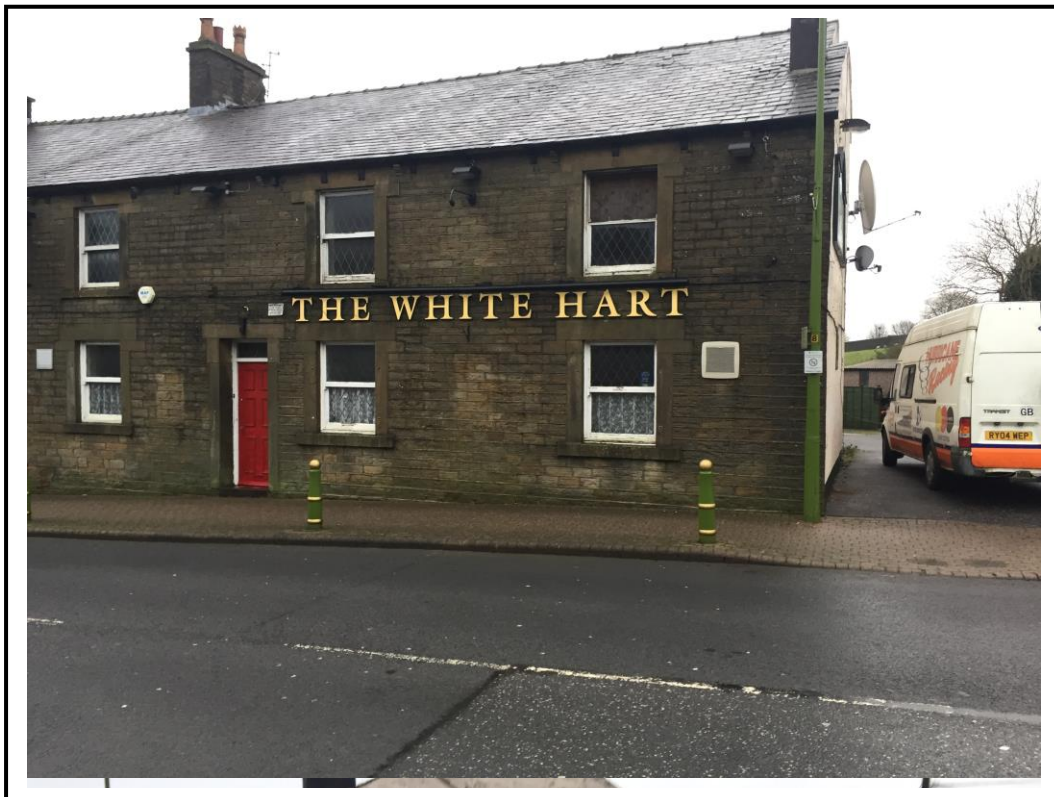
Photo 1 – front elevation of existing building
